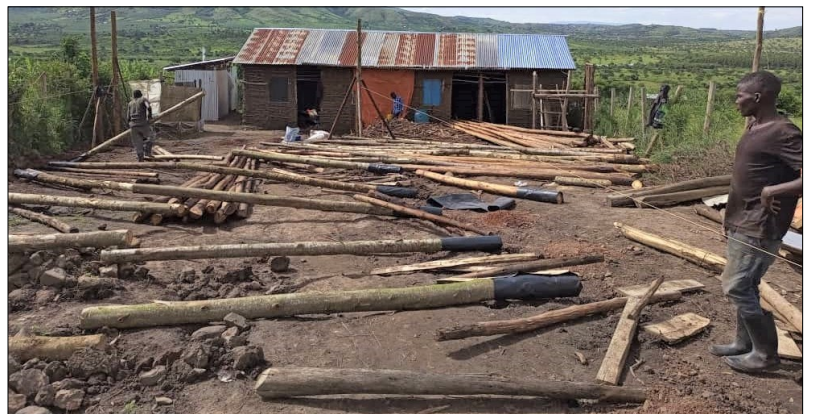
Poles being laid out into position
