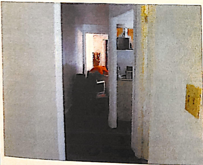
View from top of stairs to kitchen at 241 West Main St., Apt. C, Cortland, Ohio
