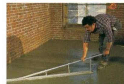
Fig. 5.2—Finishing a cellular concrete floor.
