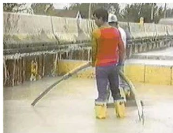
Fig. 5.1.2—Flowability of cellular concrete (video courtesy of Elastizell).
