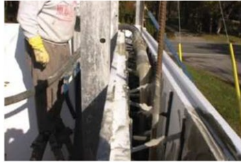
Fig. 5.1.1—Reusable formwork for a wall panel
