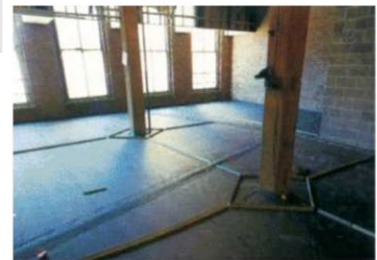
Fig. 5.2.3—Crack control strips.
