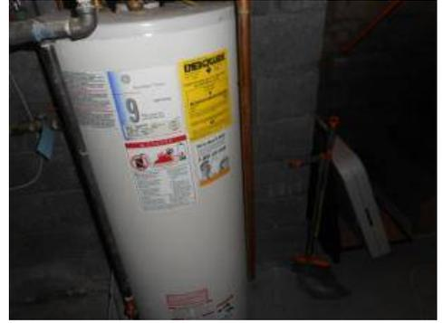
**VISUAL CONDITION/OPERATION:** The unit is operational, but the installation does not meet all of the modern recommended safety guidelines. See below for details. Electrical bonding/jumper wire not installed. Consider installing to continue ground through water tank.
