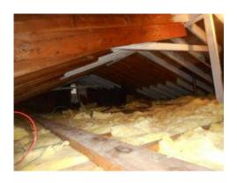
ROOF SHEATHING: Plywood where visible.
