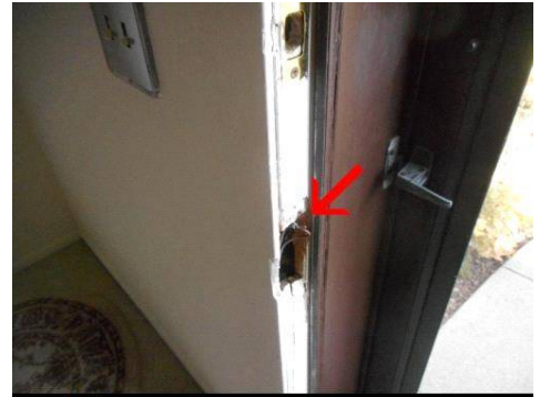
jamb damaged
