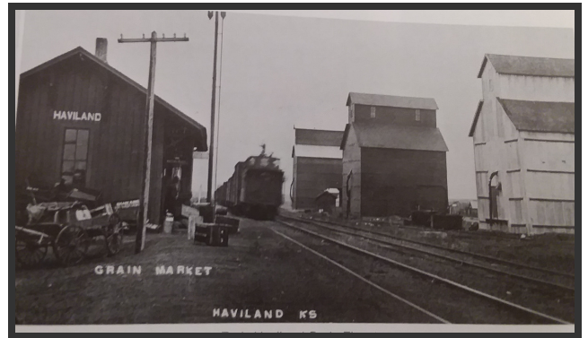
Early Haviland Grain Elevators
