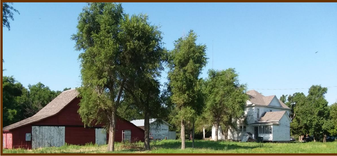
Konkel House – Back of barn, NE sides of house – 7/18/2019
