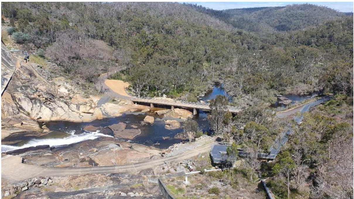
Downstream view of the Wellington Dam
