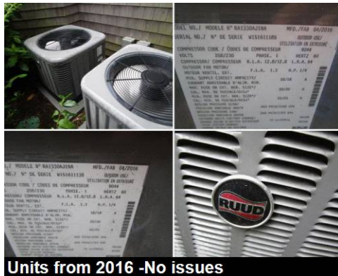
Units from 2016 -No issues
