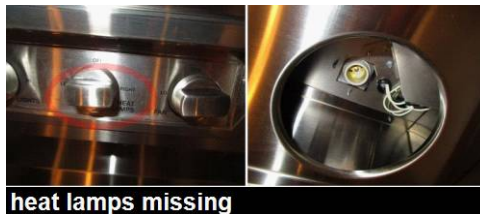
heat lamps missing
