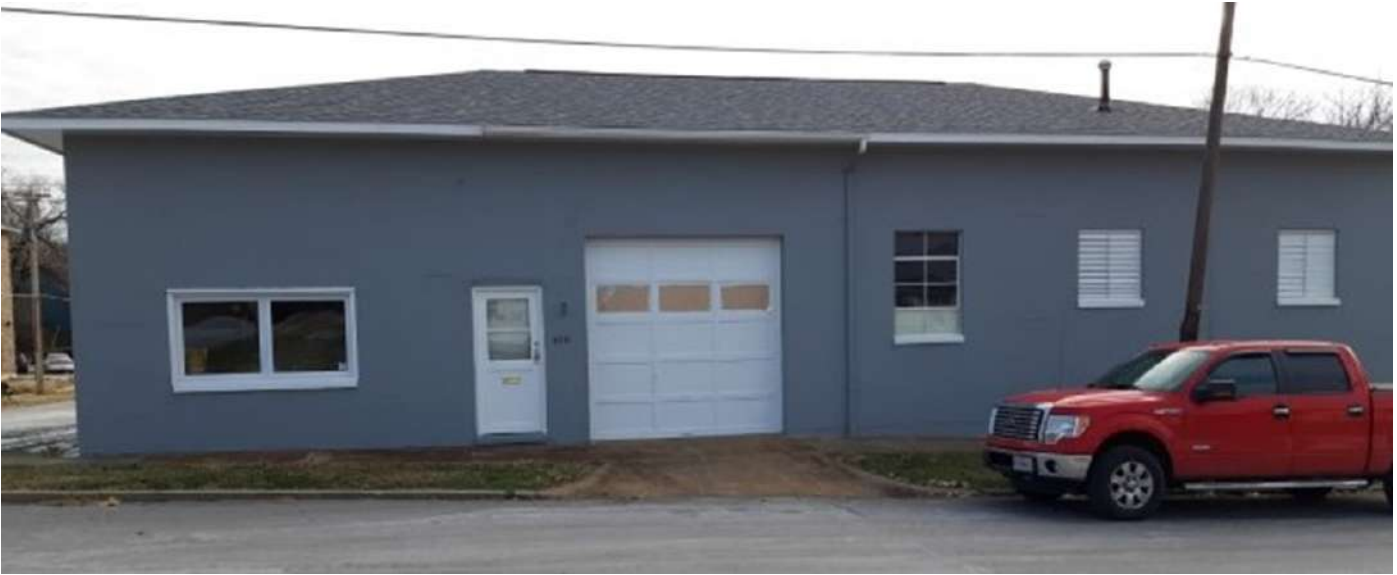
The building located at 410 N. Elm Street, Rolla, MO
