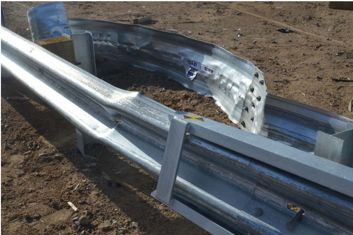
FIGURE 34. Test Article Damage
