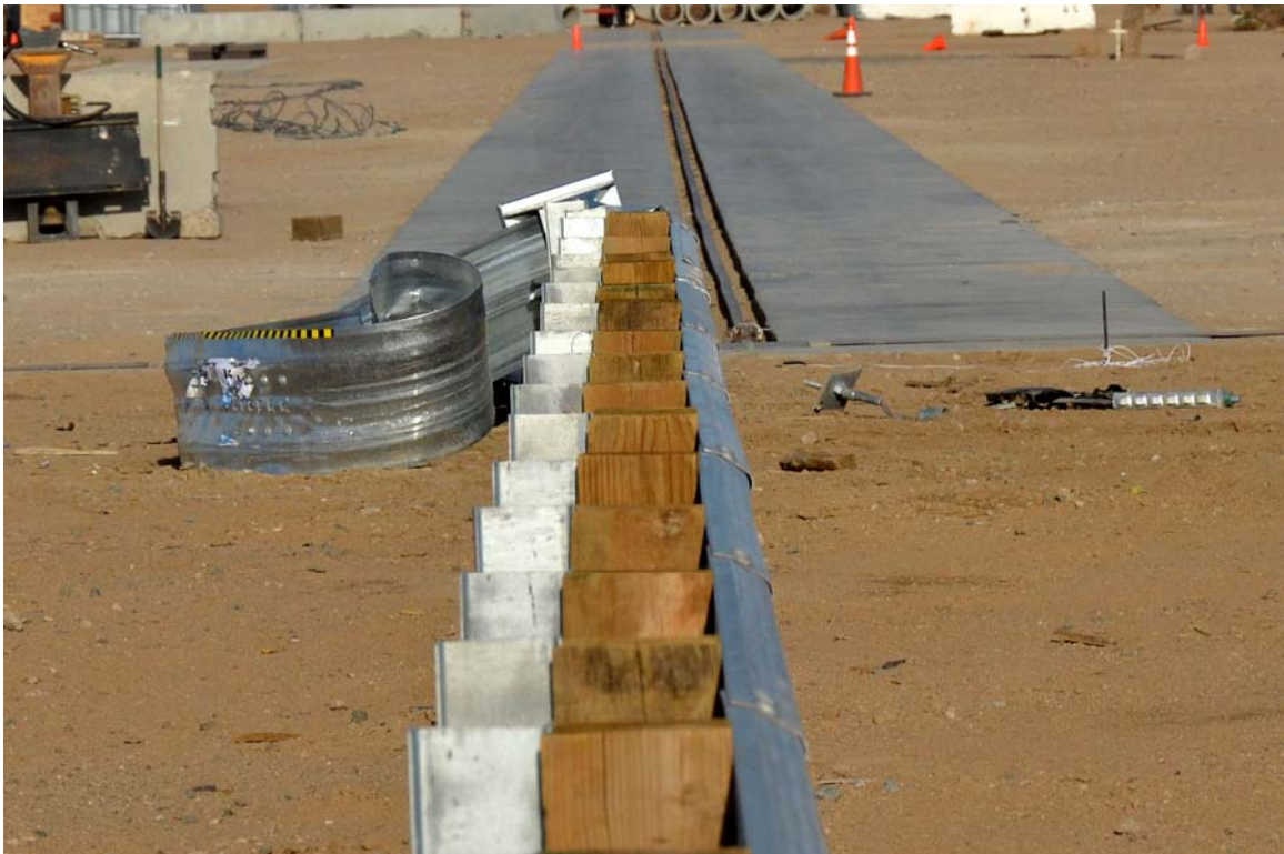
FIGURE 24. Post-Test Rear View of Test Article
