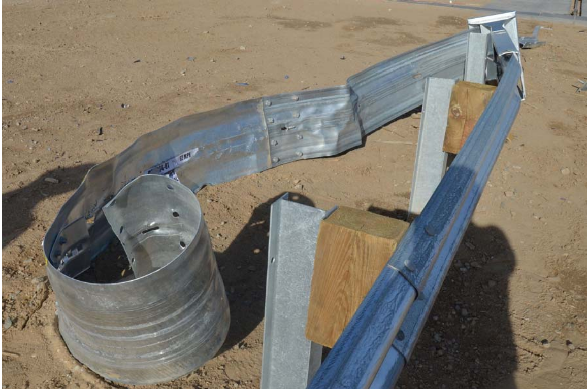
FIGURE 33. Test Article Damage
