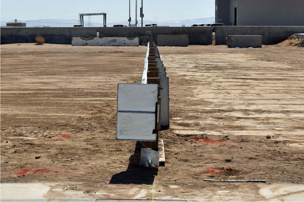
FIGURE 15. Pre-Test Front View of Test Article
