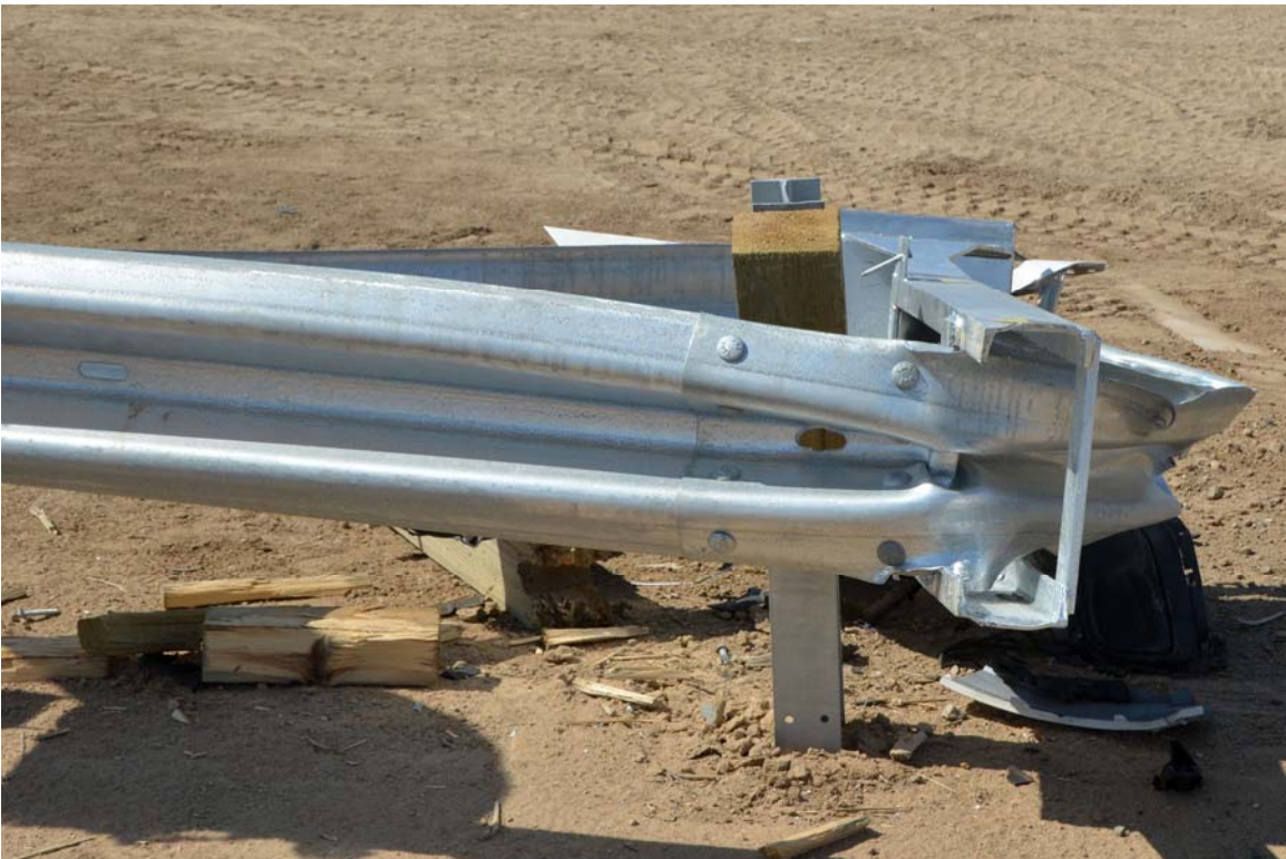
FIGURE 36. Test Article Damage
