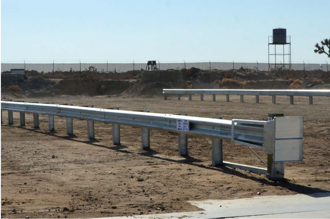
FIGURE 17. Pre-Test Right Front \frac{3}{4} View of Test Article
