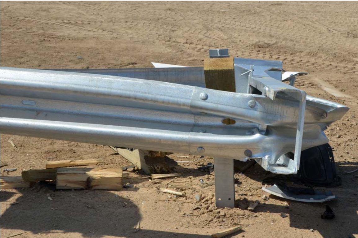
FIGURE 36. Test Article Damage
