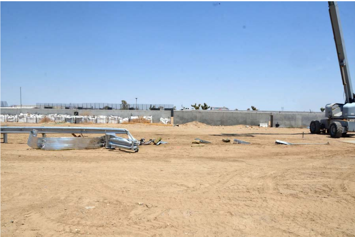
FIGURE 20. Post-Test Right View of Test Article
