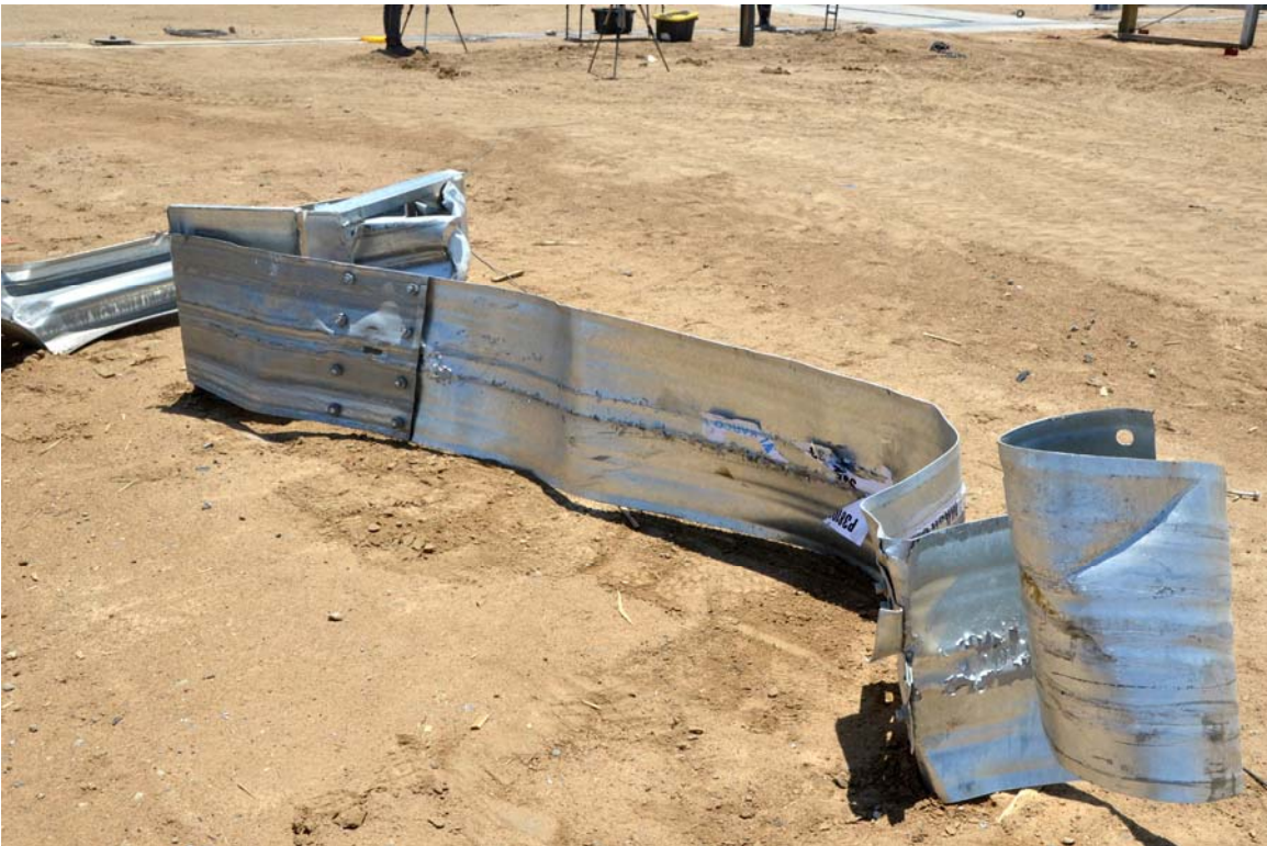
FIGURE 36. Test Article Damage
