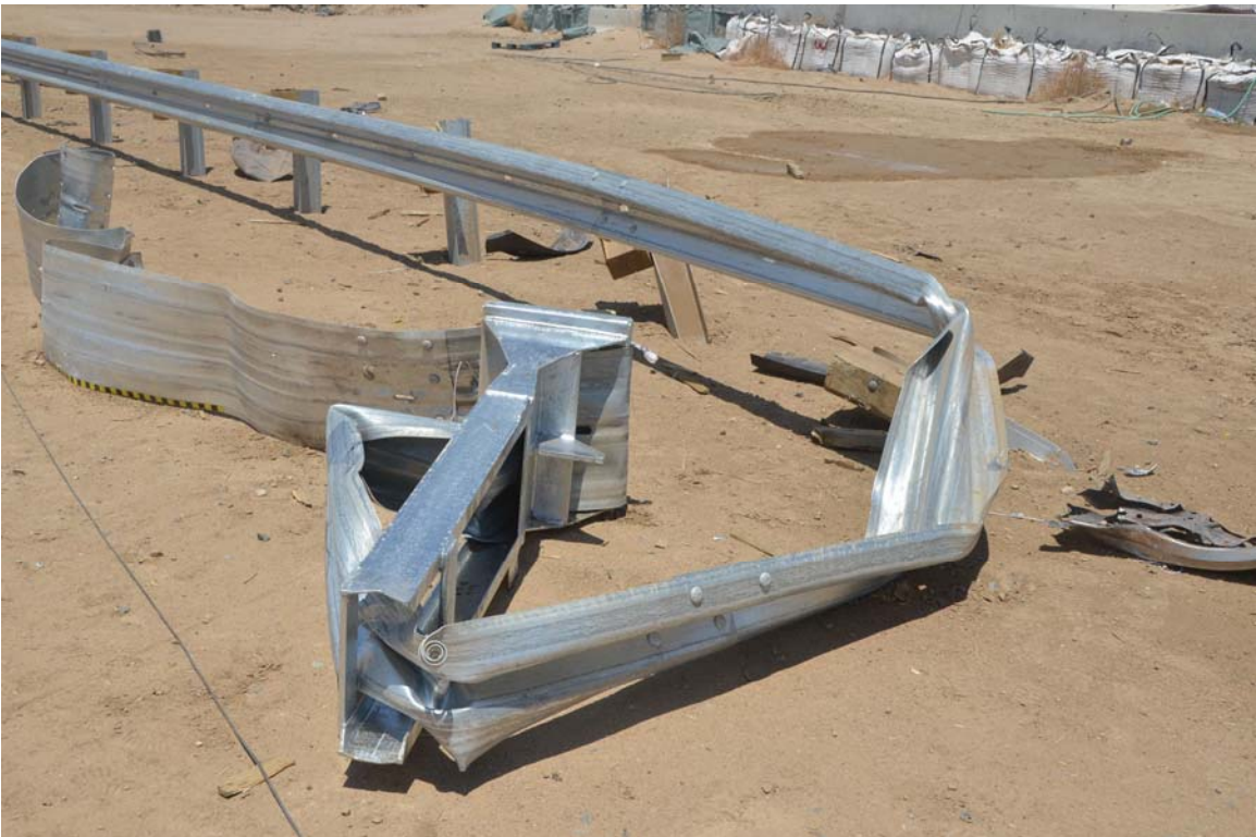
FIGURE 32. Test Article Damage
