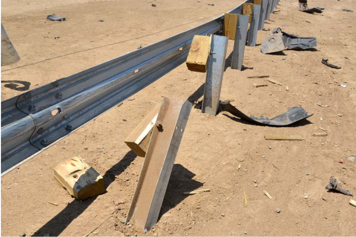
FIGURE 33. Test Article Damage
