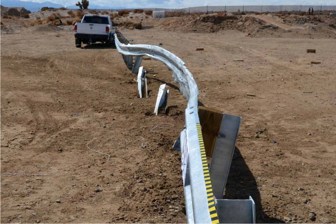
FIGURE 31. Test Article Damage
