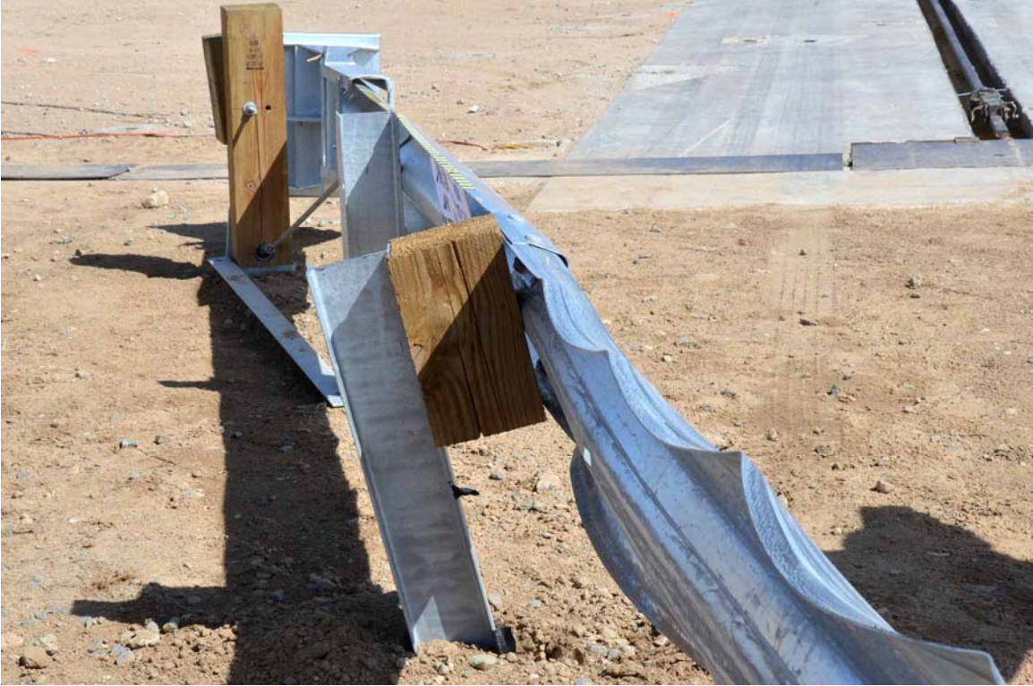
FIGURE 35. Test Article Damage
