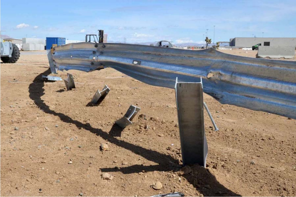
FIGURE 33. Test Article Damage
