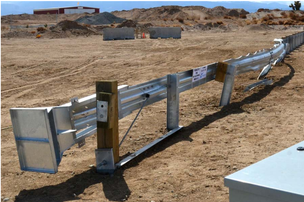
FIGURE 30. Post-Test Left Front \frac{3}{4} View of Test Article
