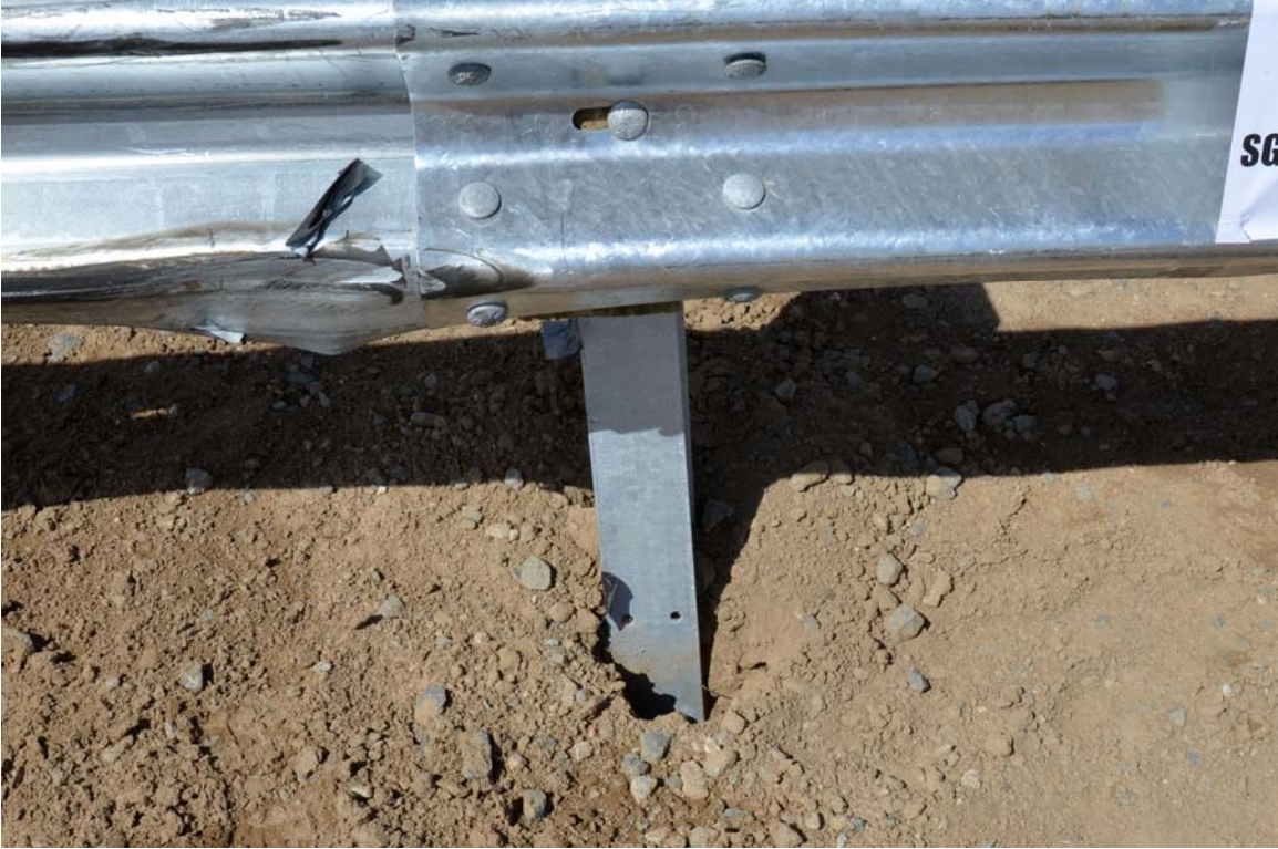
FIGURE 35. Test Article Damage
