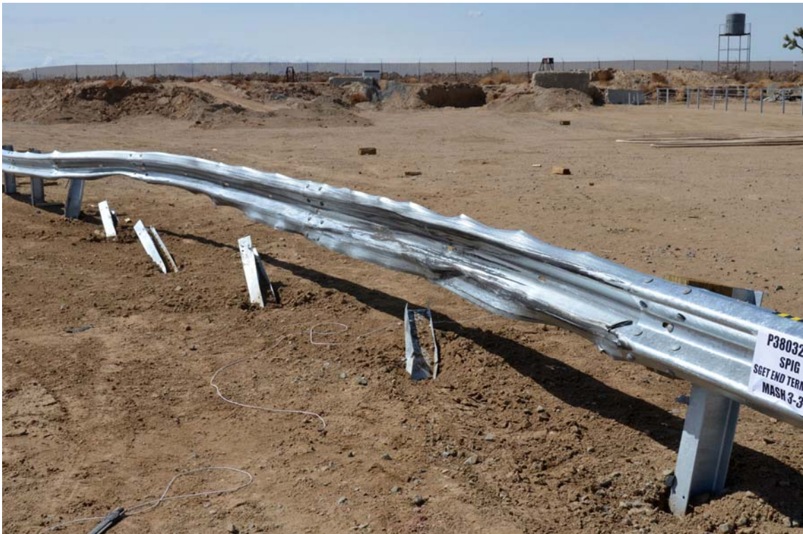
FIGURE 32. Test Article Damage
