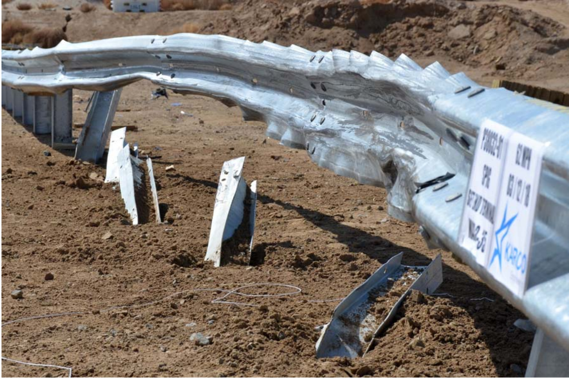
FIGURE 33. Test Article Damage
