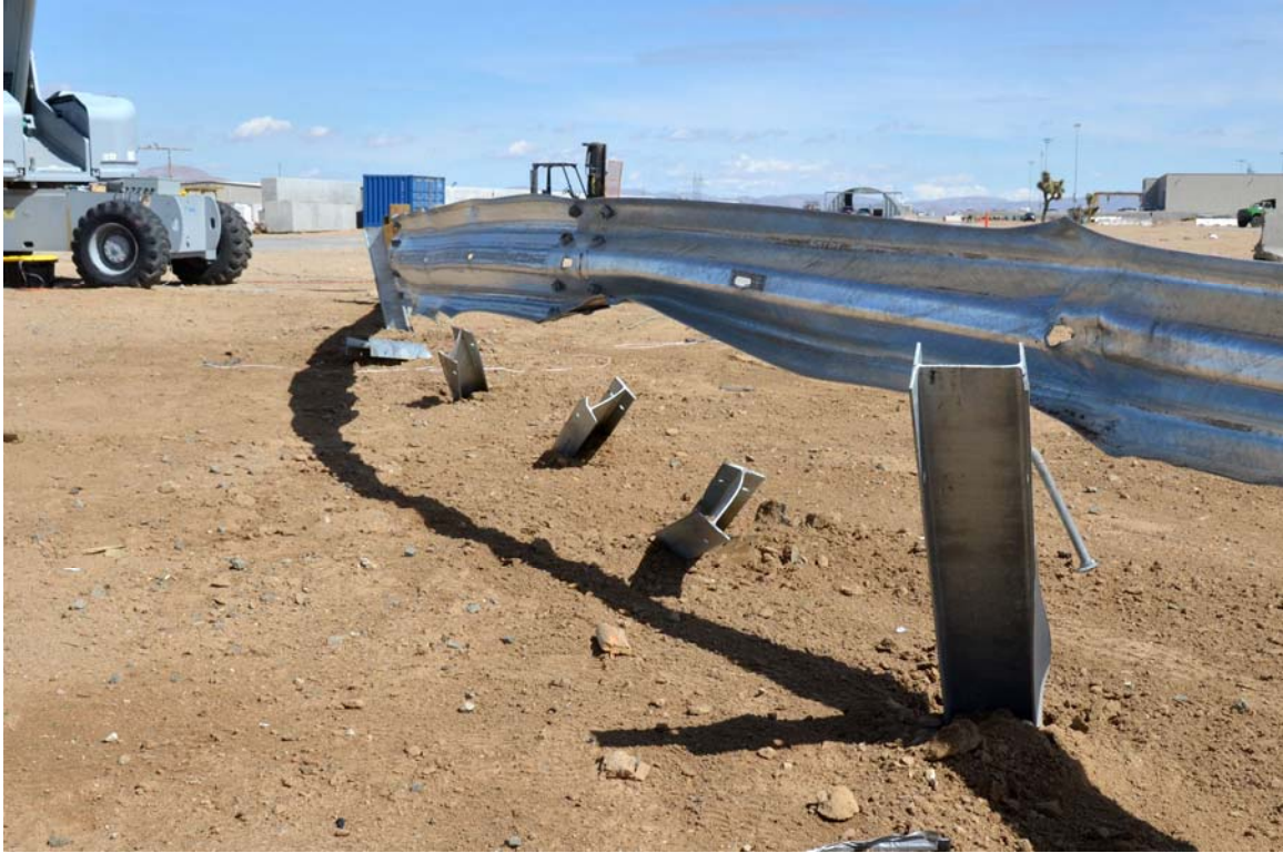
FIGURE 31. Test Article Damage
