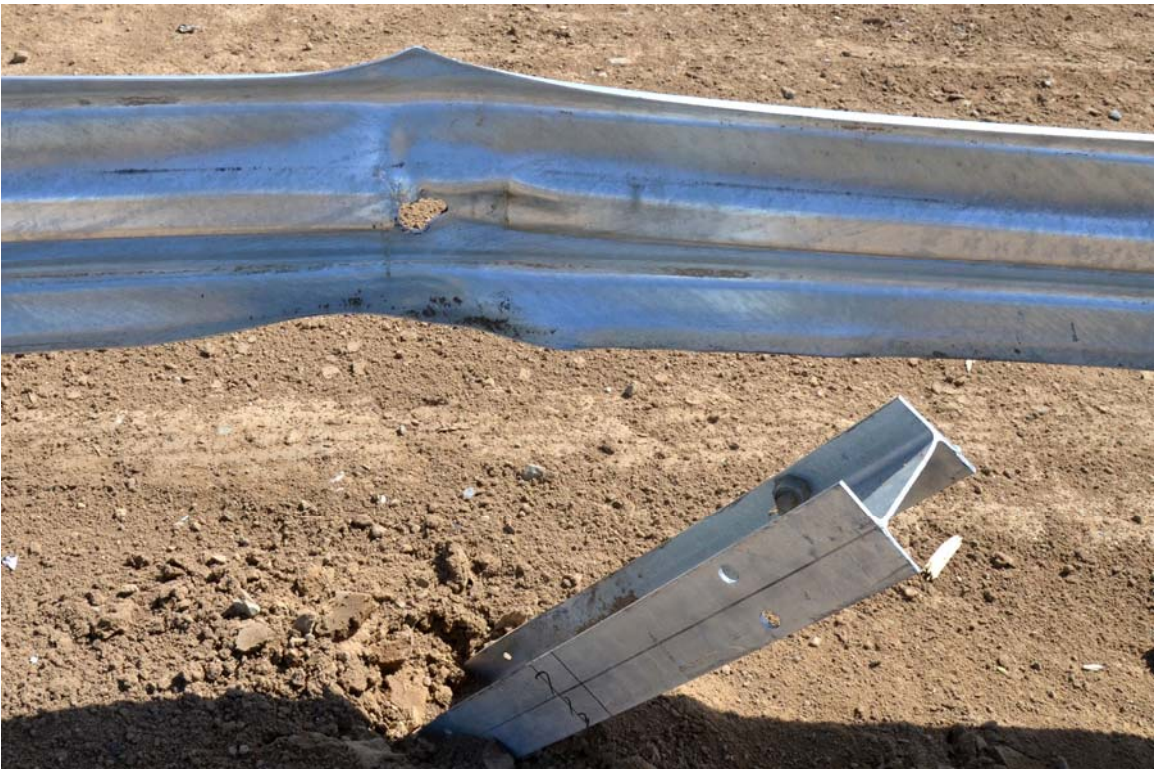
FIGURE 36. Test Article Damage
