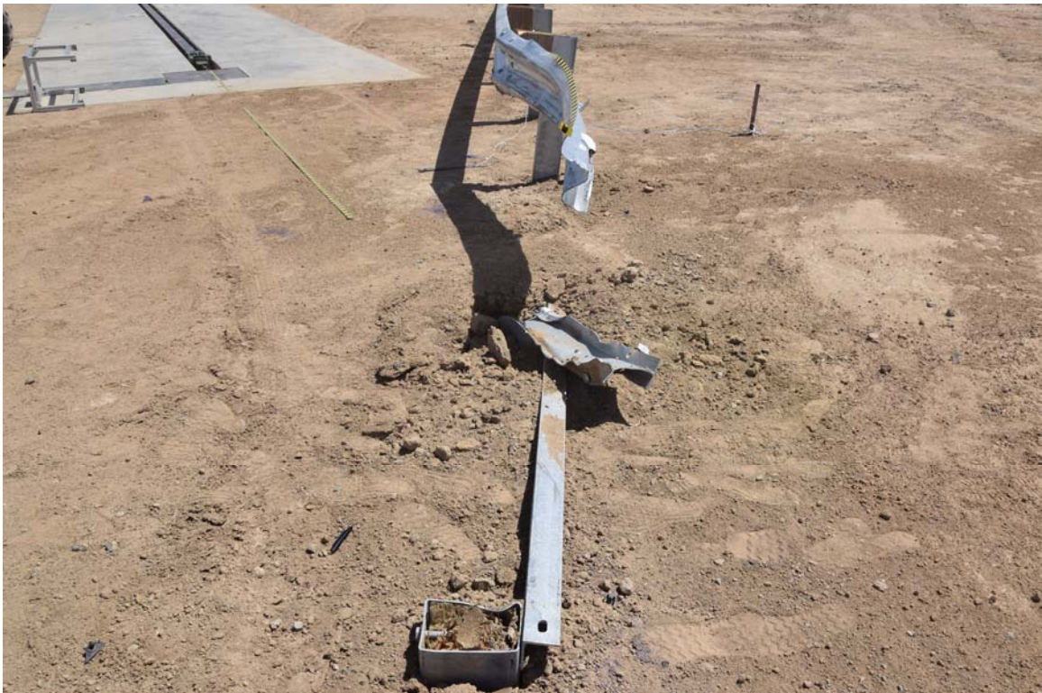
FIGURE 34. Test Article Damage
