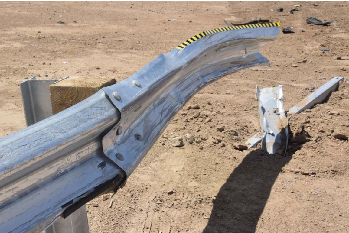
FIGURE 32. Test Article Damage
