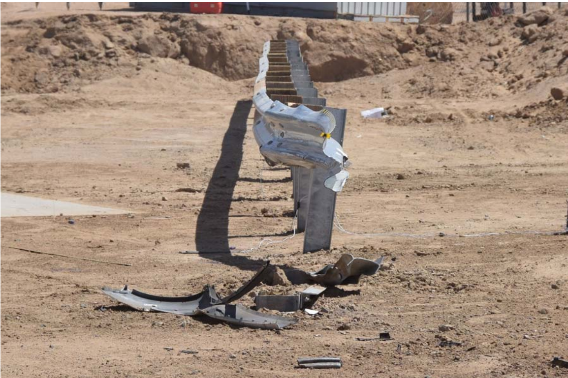
FIGURE 16. Post-Test Front View of Test Article
