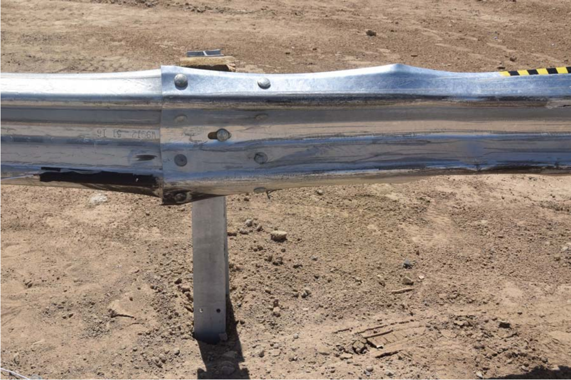
FIGURE 31. Test Article Damage
