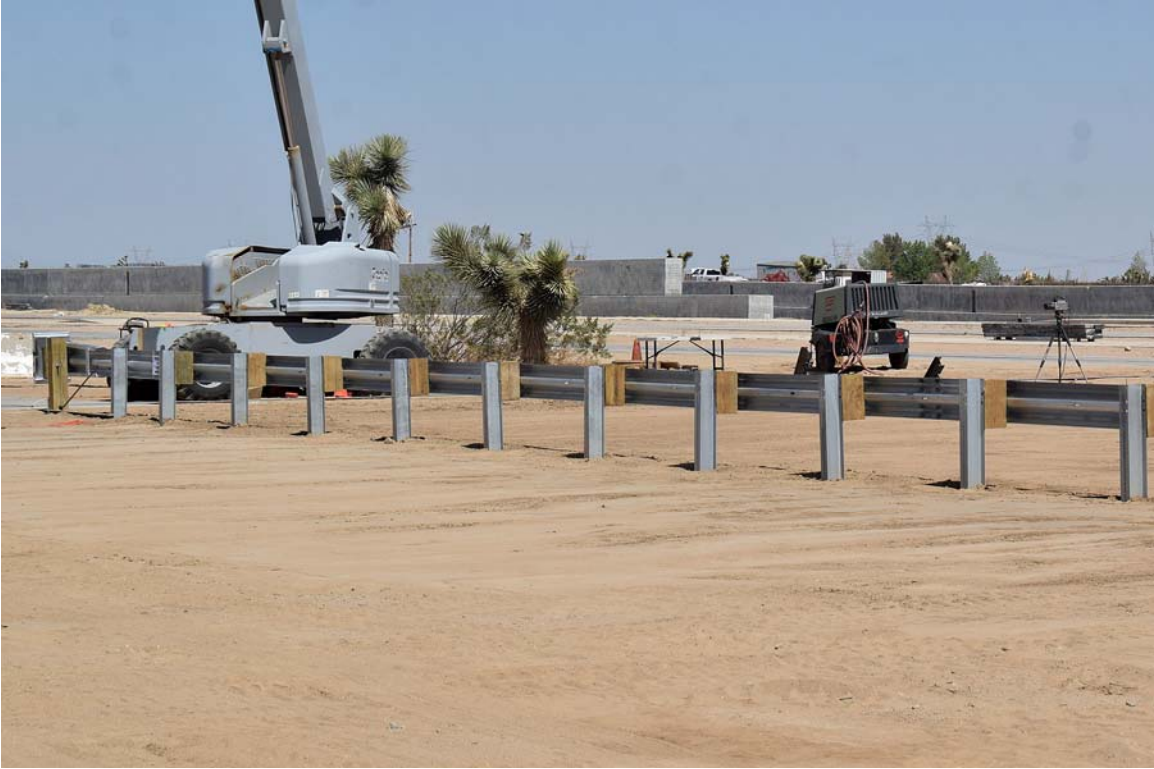
FIGURE 25. Pre-Test Left Rear \frac{3}{4} View of Test Article
