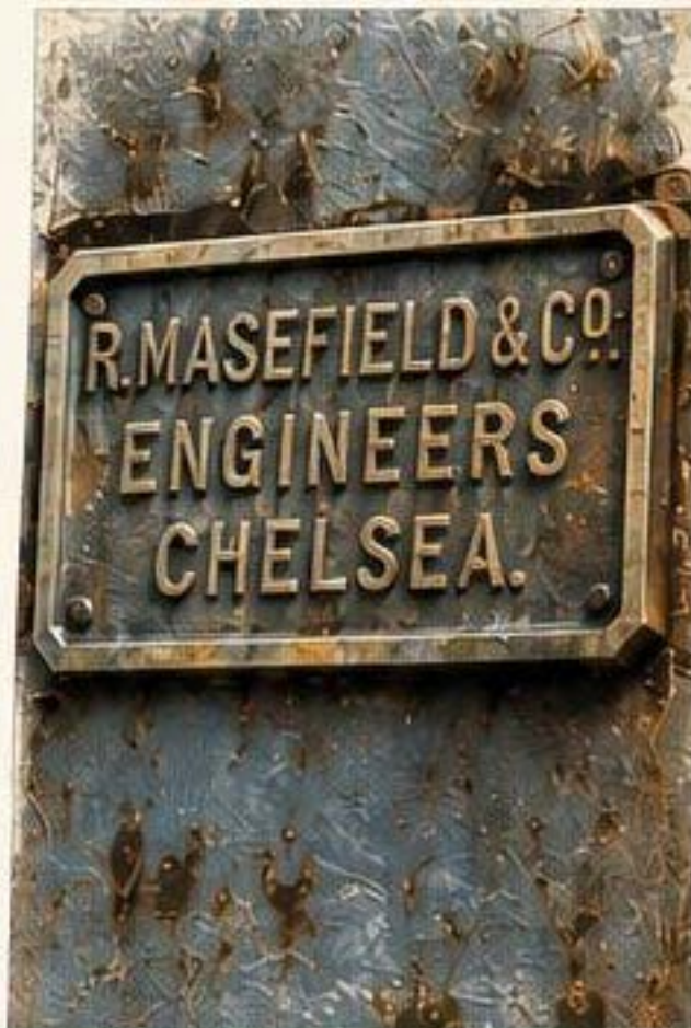
The maker's plate on Little Hereford footbridge LH19
