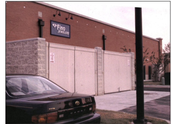
The top photo shows appropriate trash enclosure constructed of broken-face block and with wood gates. The photo below shows a pedestrian walk-through from parking to the street. Pedestrian connections in the Downtown District should be designed with attention to detail to welcome visitors.
