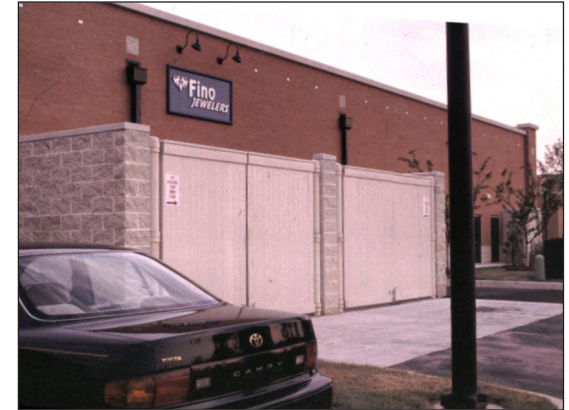
The top photo shows appropriate trash enclosure constructed of broken-face block and with wood gates. The photo below shows a pedestrian walk-through from parking to the street. Pedestrian connections in the Downtown District should be designed with attention to detail to welcome visitors.
