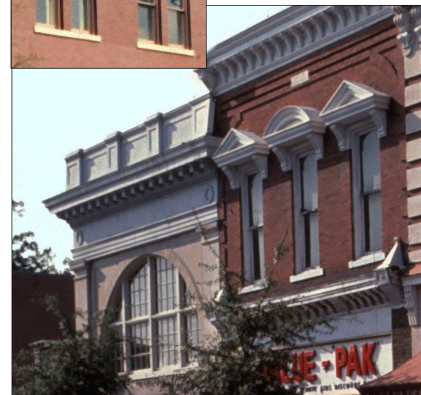
Windows add not only light, but interest. Note the various types of trim and moldings on the cornices and windows of these buildings
