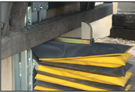
Hydraulic operation to raise the restraint and engage the Rear Impact Guard.
