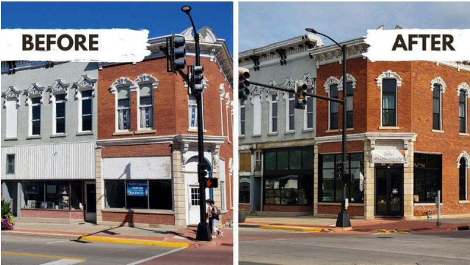
Before and after facade improvements | Source: Independenceia.gov
