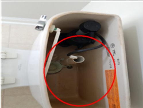
Toilet tank floater is missing from this toilet. A licensed plumbing contractor should be consulted for a complete evaluation and to make necessary repairs.
