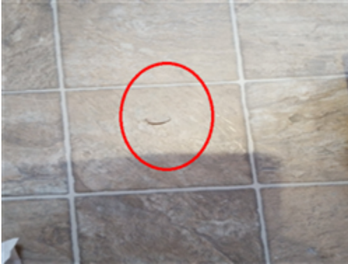
Damaged vinyl flooring.
