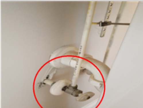
Water supply lines are loose. This condition can result in water leaking into the wall areas. A licensed plumbing contractor should be consulted for a complete evaluation and to make necessary repairs.
