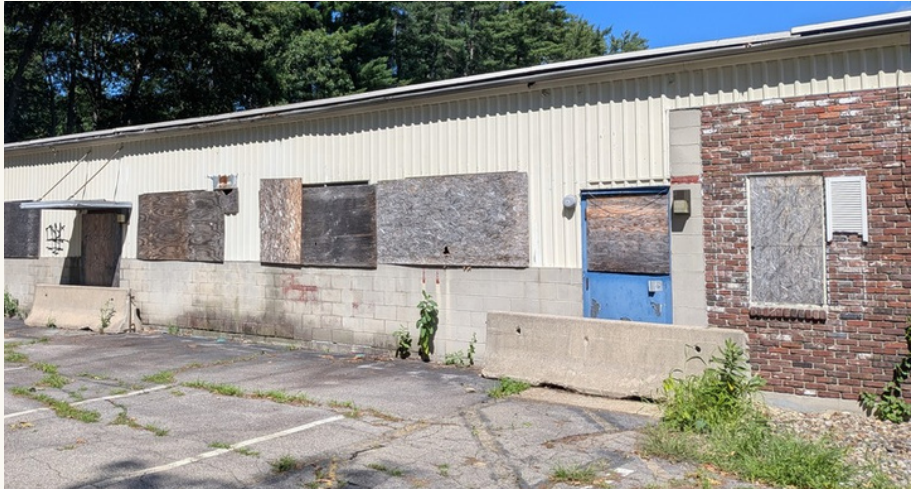
The east side of the Elm Street building today, covered in graffiti. Milford Historian photo.
