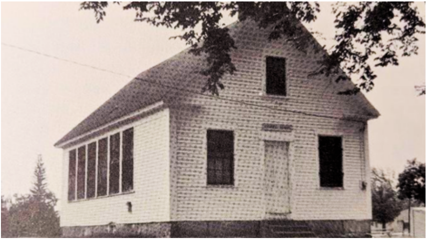
Above: The Laurel School in 1972. Photo: Historic Building Conditions Assessment Report.
