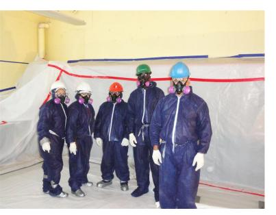
PCBs were added to caulk and elastic sealant materials, particularly from 1950-1977. When caulk with PCBs is disturbed, it may produce dust that contains PCBs. The SCA has developed and implemented stringent dust control practices to minimize the potential exposure to PCB-containing dust during construction.
