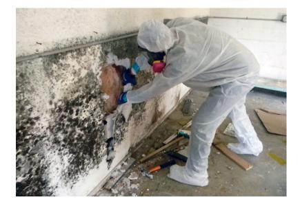
The SCA's environmental consultants assess potential mold growth, water damage, or musty odors in the school. Equipment is employed to view spaces in ductwork or behind walls, as well as to measure moisture in building materials that may encourage mold growth.
