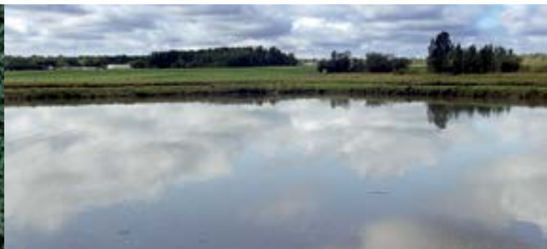
Buck Creek wastewater lagoon Cell 1
