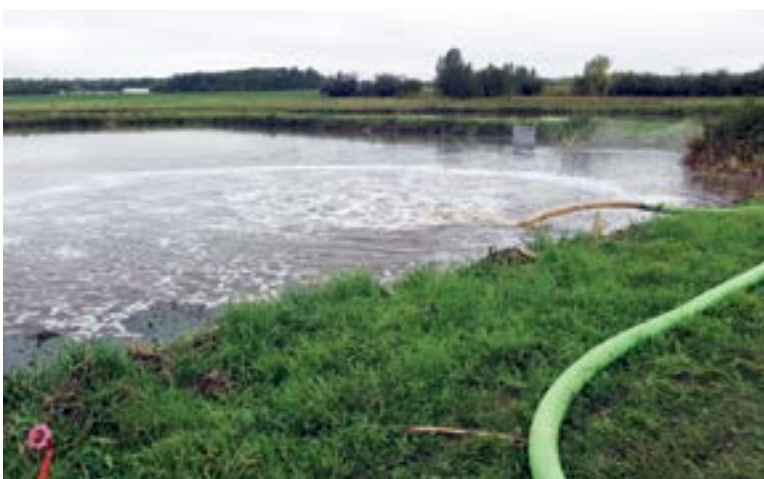
Applying Waste Go to Cell 1
