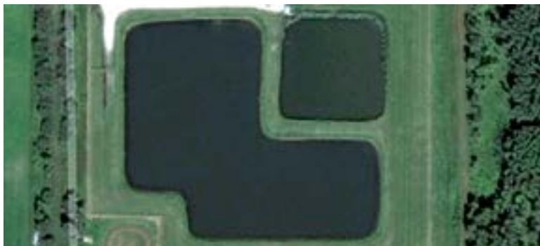
Buck Creek wastewater lagoon aerial photo
