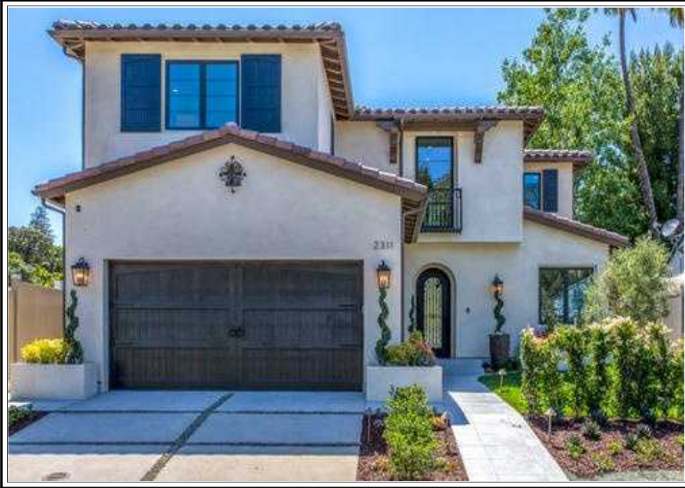
FRONT OF SUBJECT PROPERTY 2311 Beverwil Dr Los Angeles, CA 90034
