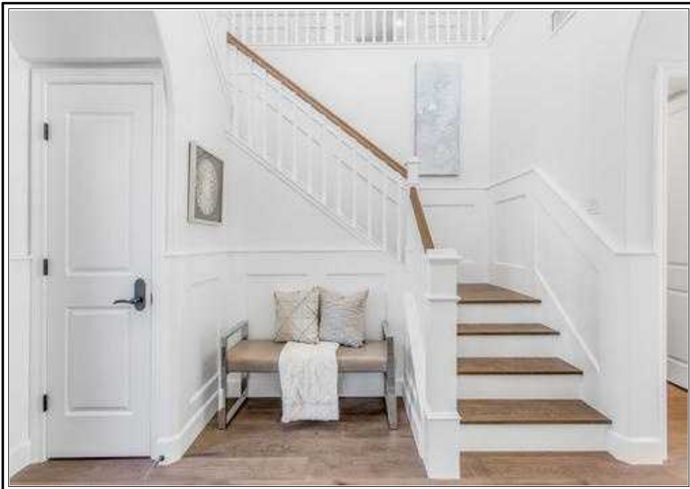
CUSTOM WAINSCOTING & HARDWOOD FLOORING DETAIL IN ENTRY
