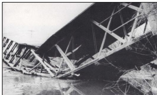
On August 31, 1977, a trucker tried to drive through Blacklick Bridge with a load that was *twelve tons over* the 5-ton limit. Today the 89-year-old bridge still lies broken in the stream; the road is closed to traffic while a settlement is being discussed; and we have been robbed of a once-handsome, useful emblem of our past.
