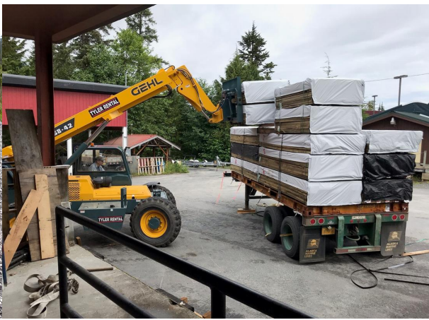
Mountain View Manor Boardwalk materials have arrived. Construction to begin this fall.
