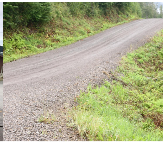
Summer work on the US Forest Service Grading and Brushing project.
