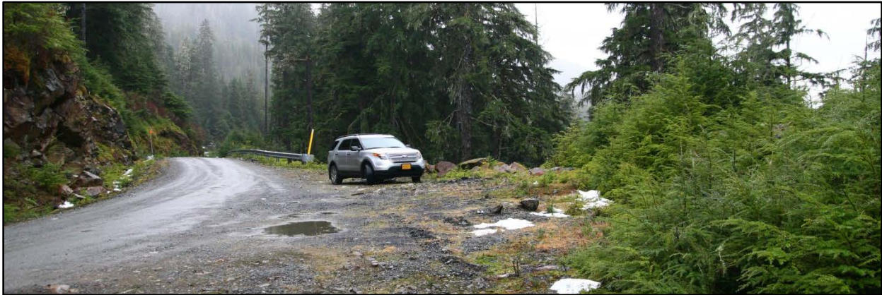
Scenic Overlook Project on the Cabin Creek Reservoir Road
