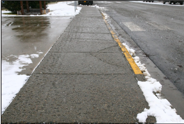
Photo of Petersburg School District's sidewalks that need reconstruction.
