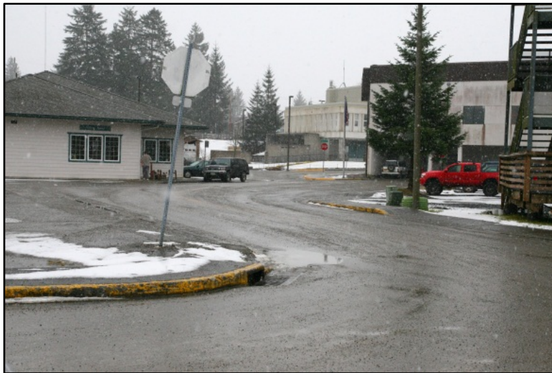
3,300 feet of North Harbor existing sidewalks need reconstruction
