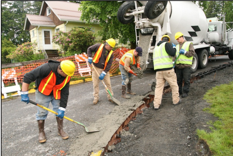
In house, PIA construction crew, working on the First Street Sidewalk Project.
