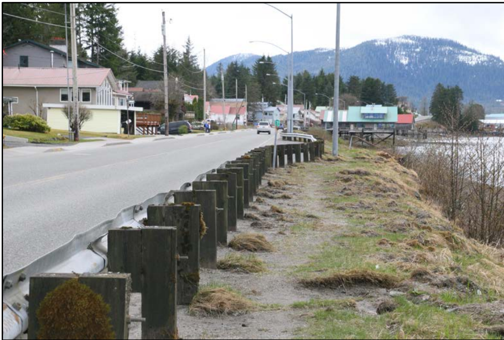
Existing North Nordic road, bike path will be on the water side of this picture.
