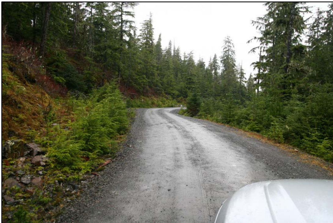
Cabin Creek Access Road, narrow 12 foot wide with limited sight distance
