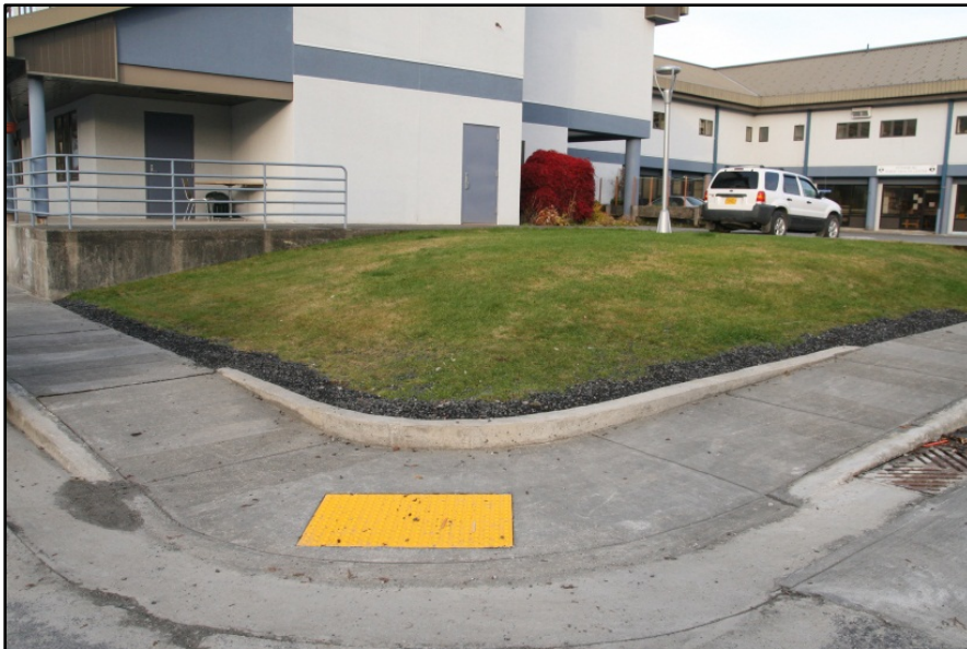
First Street Sidewalk reconstruction in front of the Petersburg Medical Center in 2011.
