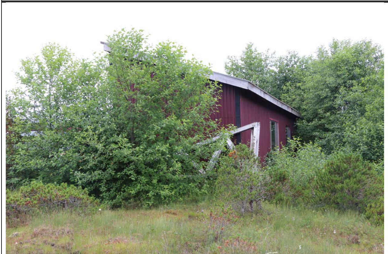
VIEW OF TTP STORAGE BUILDING TO BE DEMOLISHED – EAST SIDE
