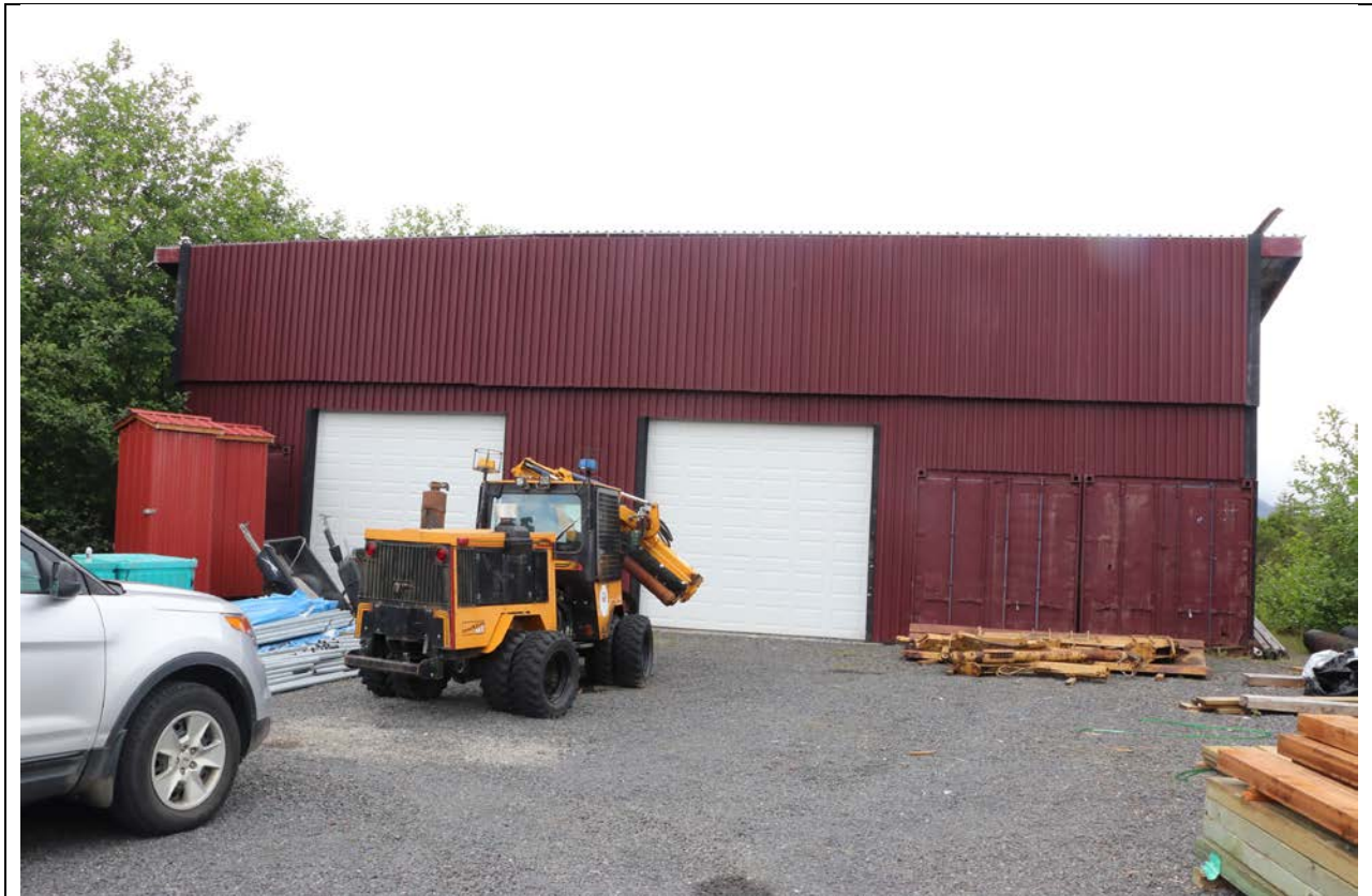
VIEW OF TTP STORAGE BUILDING TO BE DEMOLISHED – SOUTH SIDE
