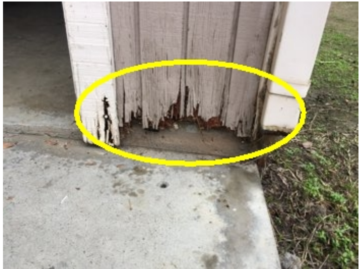
West of garage man door
