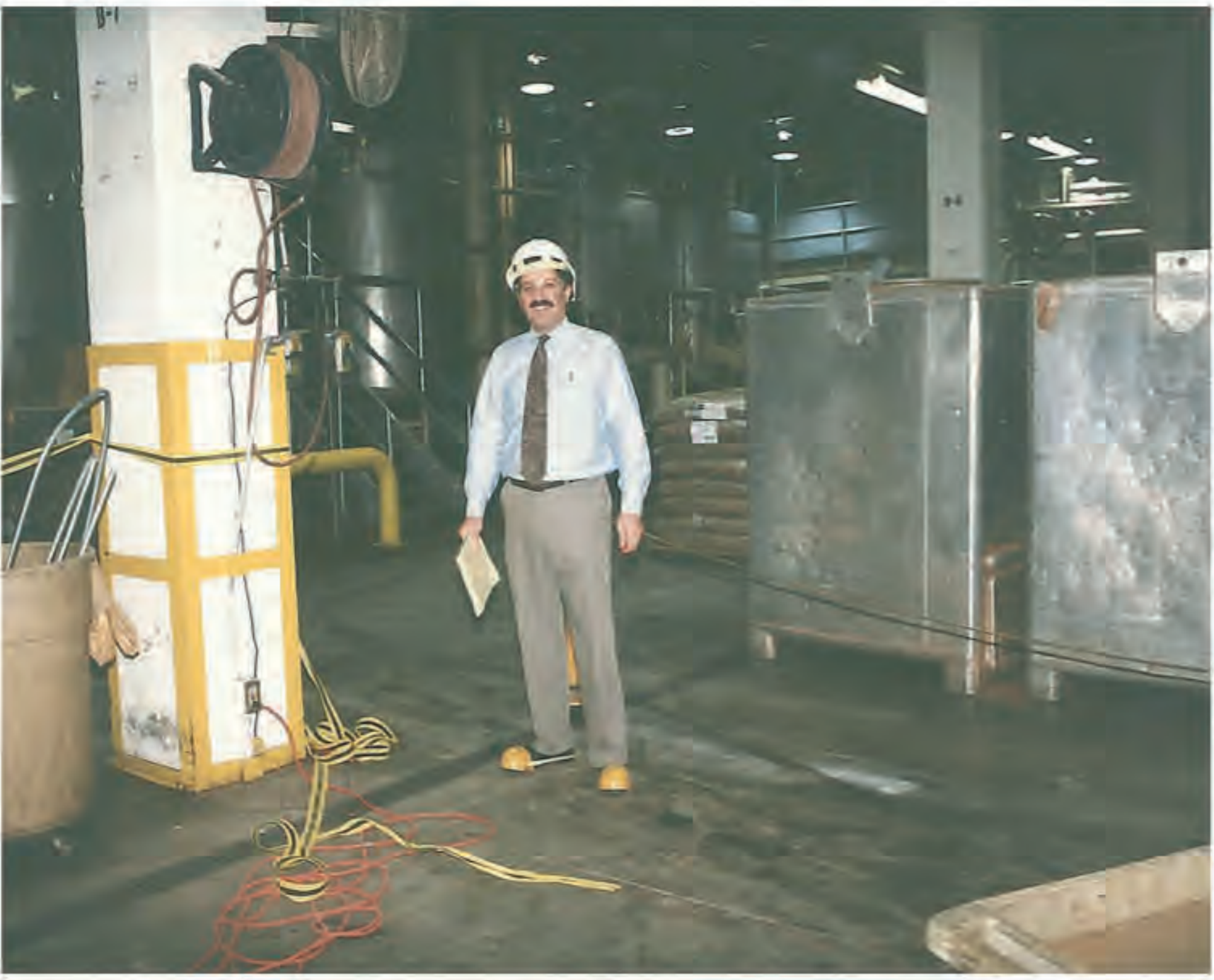
Tim Bonerb on-site during the installation of two (2) 150,000 lbs. sugar silos for Phillip Morris (Marlboro)
