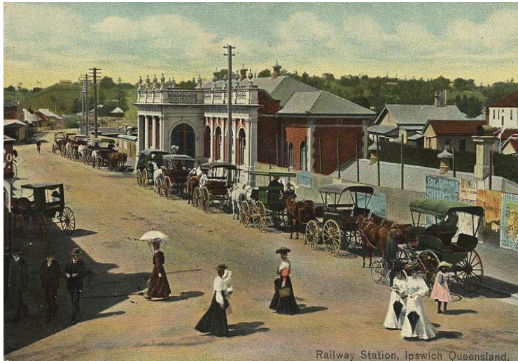
Railway Station, Ipswich Queensland.
