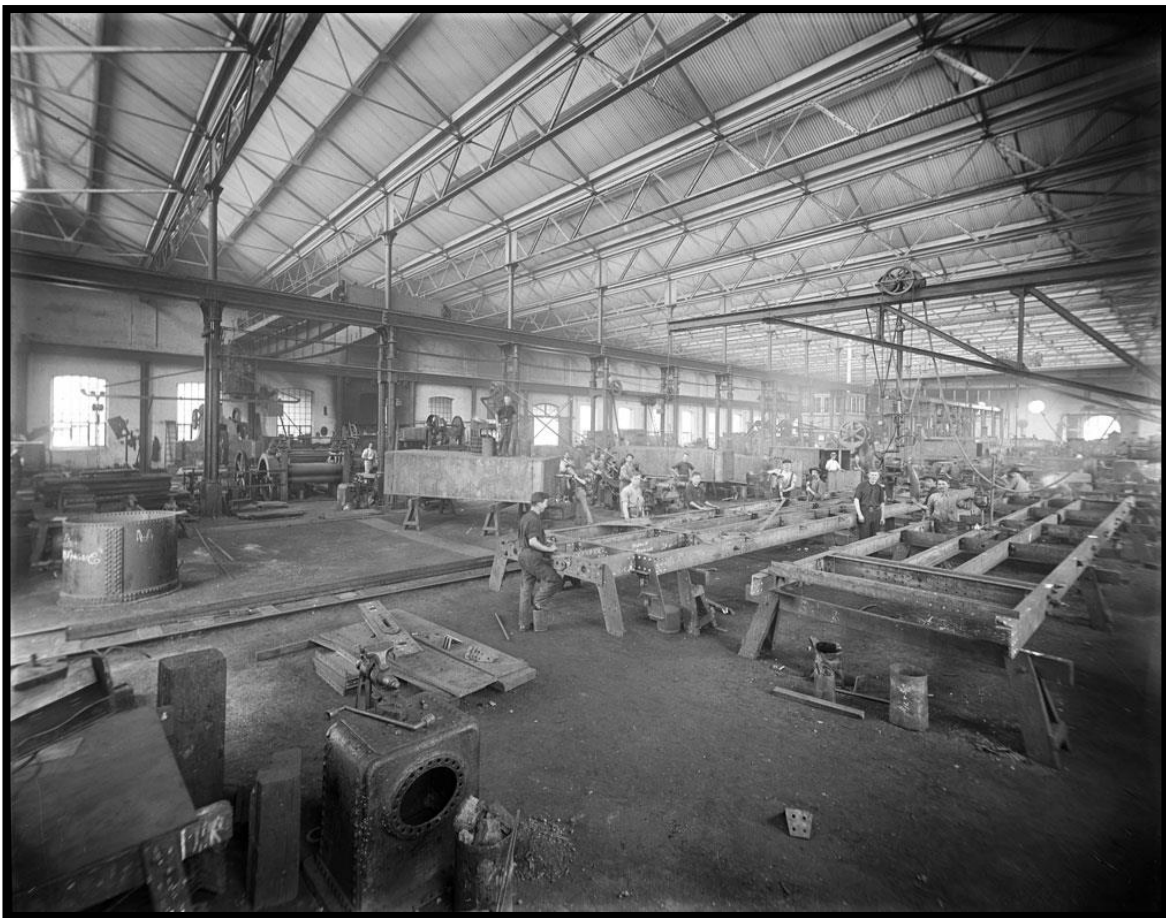
Interior of boiler shop, Ipswich Railway Workshops
