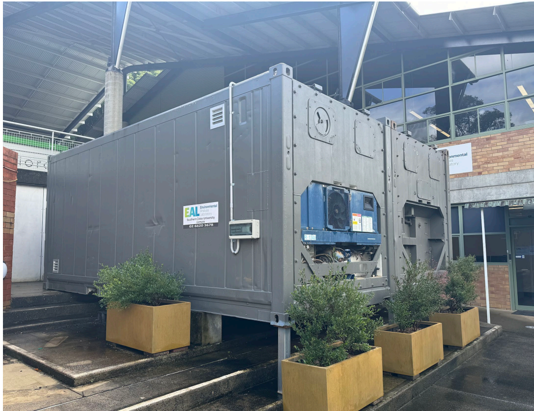
2 x 20ft insulated containers – converted into Air Dry Ovens
