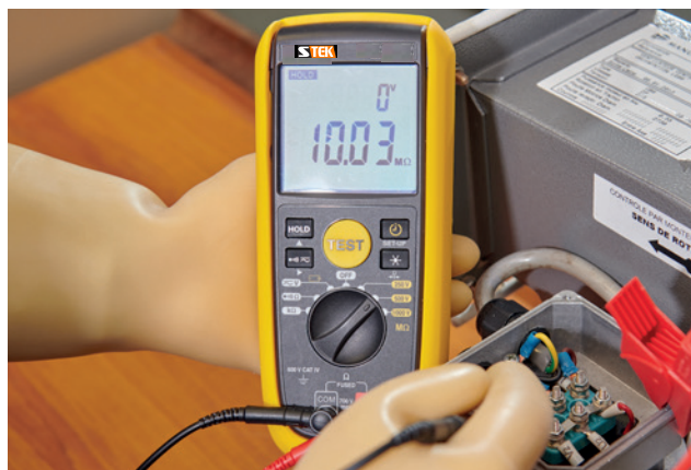
Preventive maintenance on a motor
