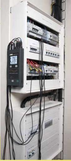
implemented are sufficient and, above all, to accurately measure any savings achieved. The monitoring by the PEL100 provides the recordings which will be compared with the reference.
