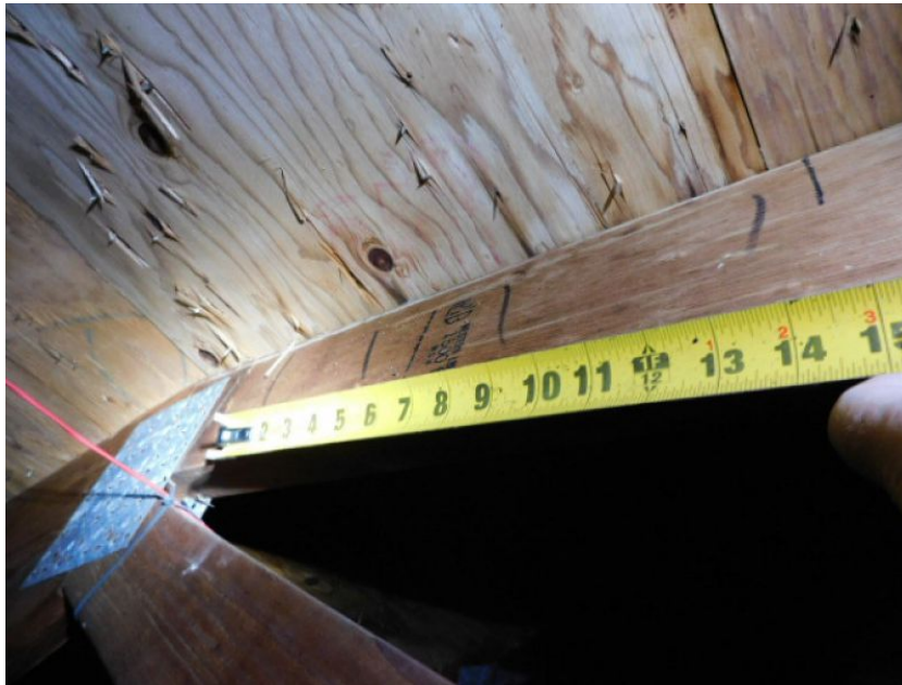
1/2" Deck Thickness Confirmed
