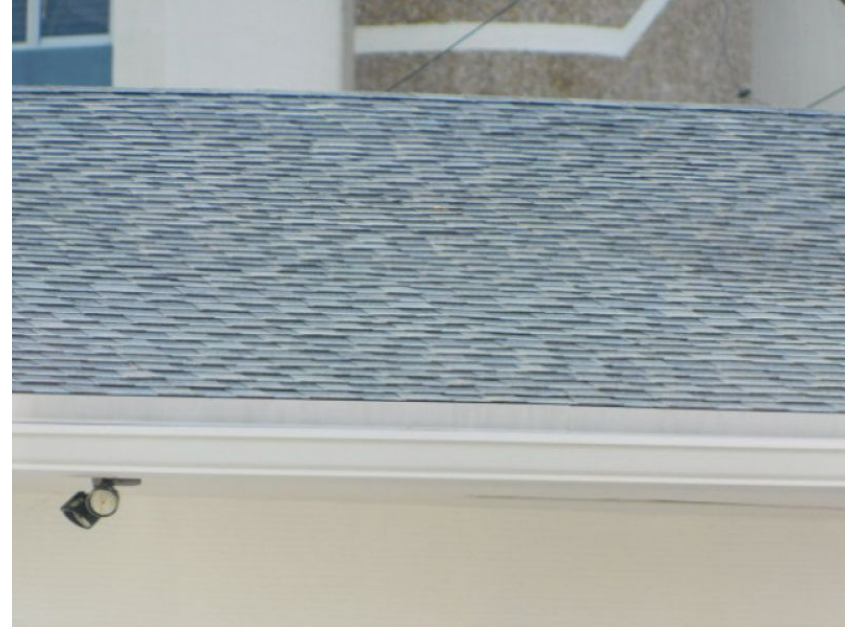
Architectural/Dimensional Shingle Roof Covering
