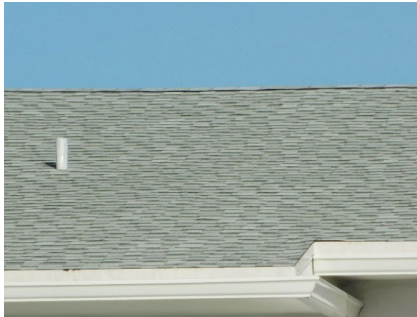
Architectural/Dimensional Shingle Roof Covering
