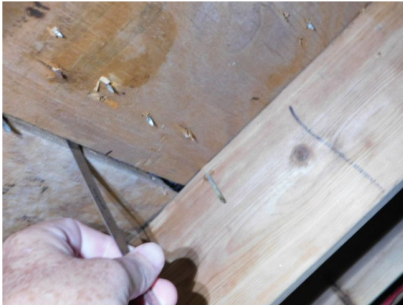
1/2" Deck Thickness Confirmed
