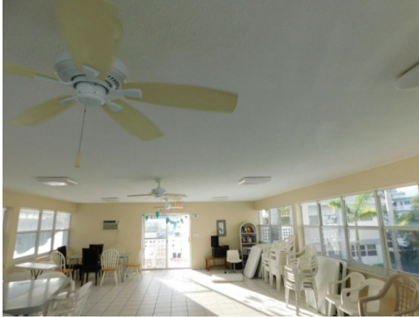
Attachment Unknown due to No Attic Access
