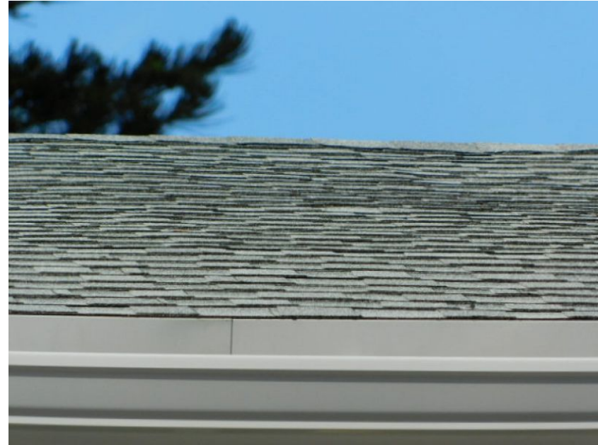
Architectural/Dimensional Shingle Roof Covering
