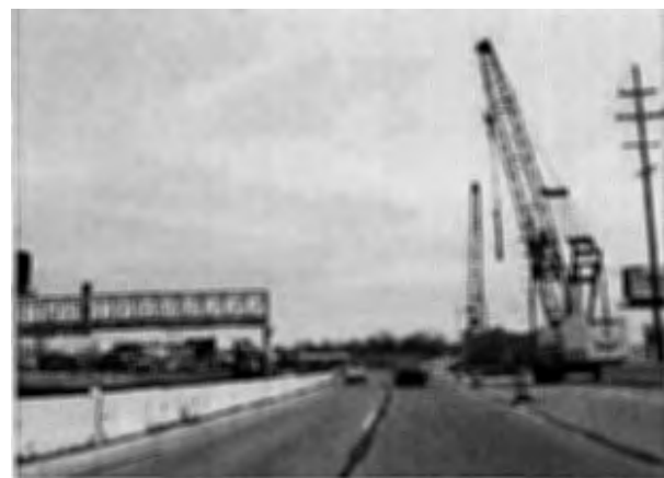
Construction of the bridge over Telegraph Road was completed in 2011.
