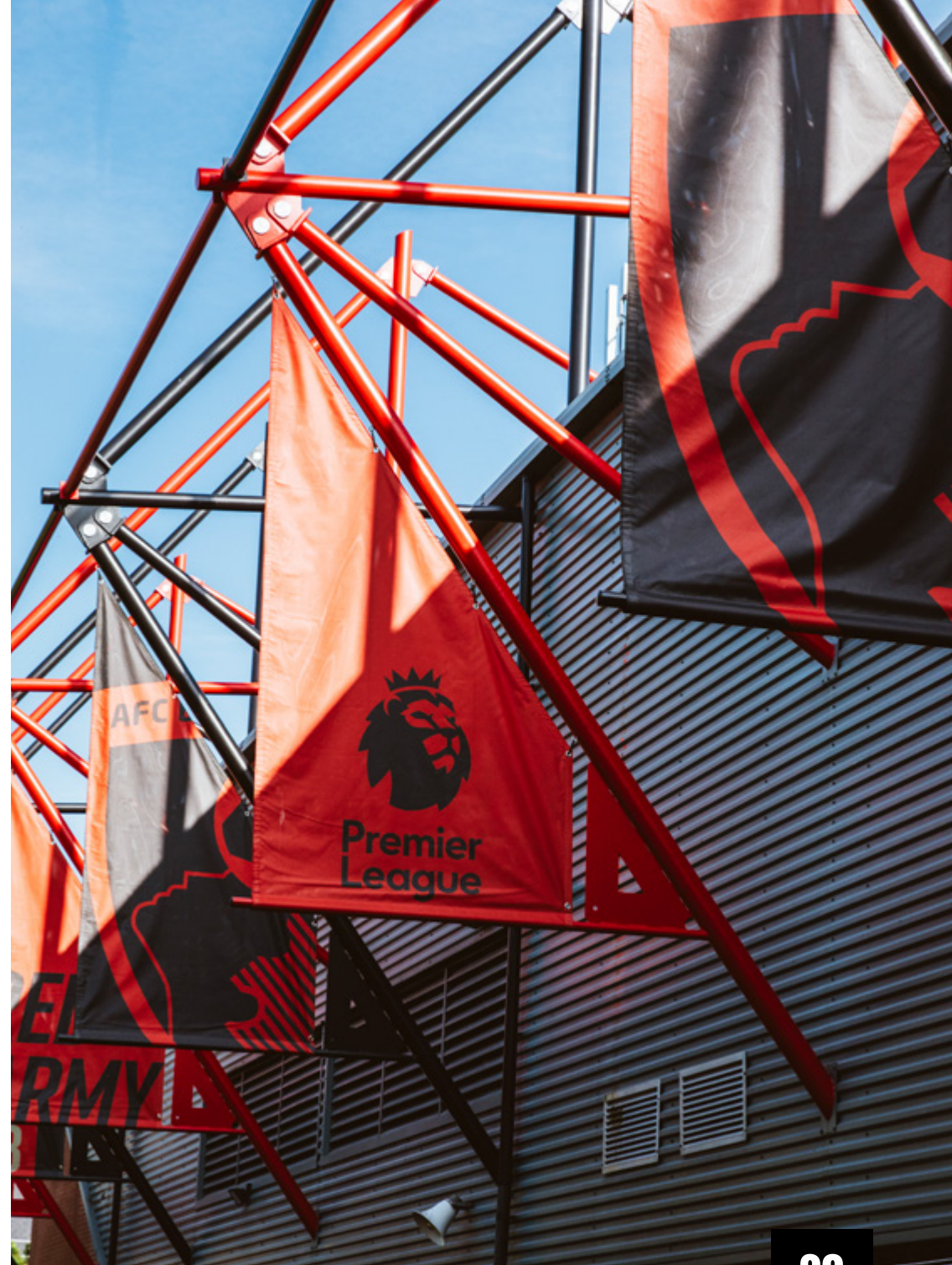
Photo: Vitality Stadium exterior
